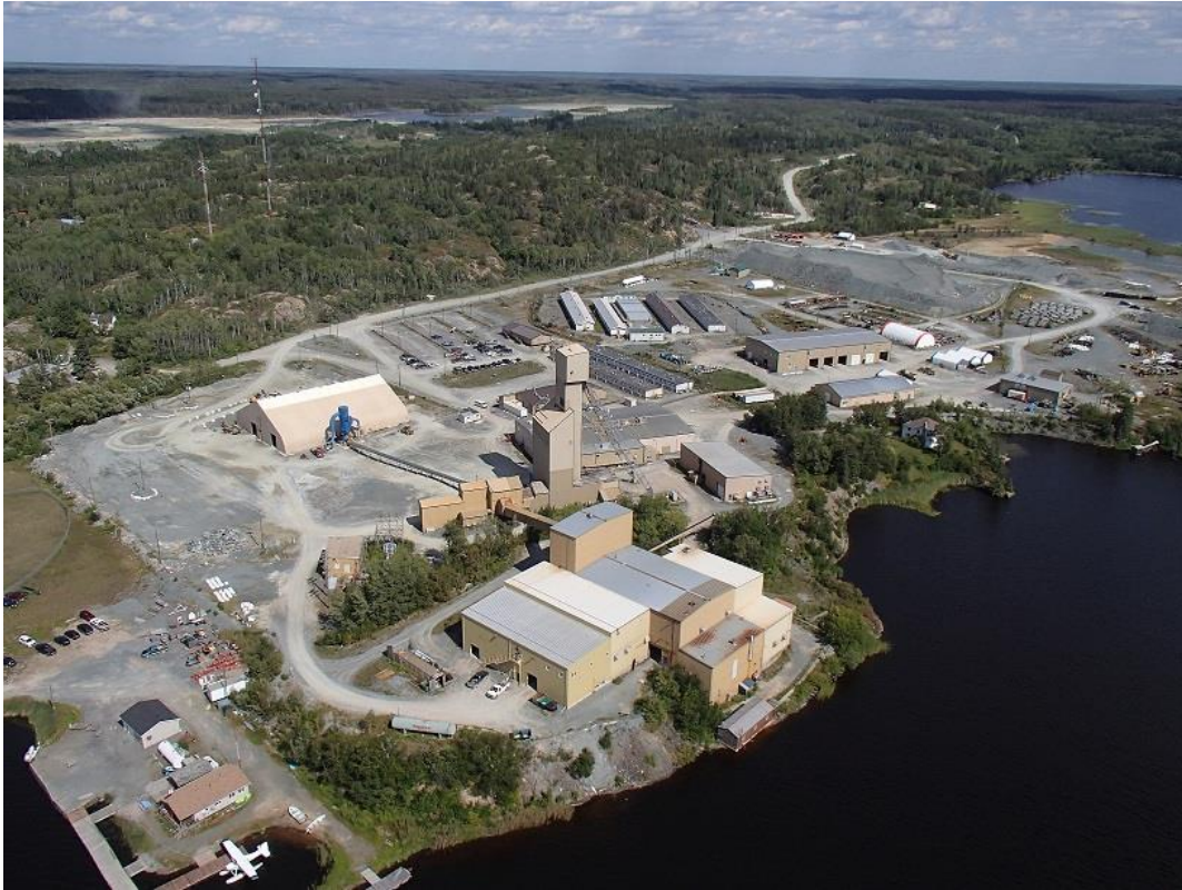
Aerial view of True North mill complex
