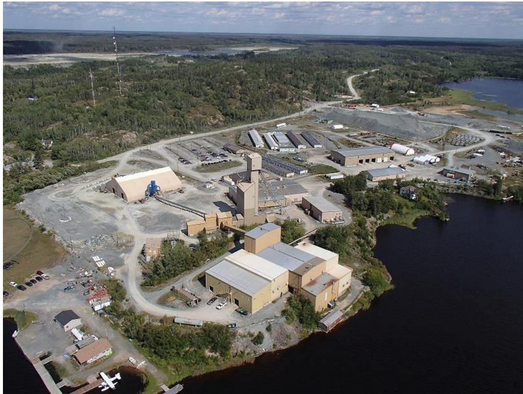
Aerial view of True North mill complex
